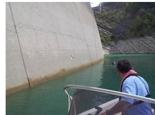
Fig. 3: Application of marker on the upstream face
